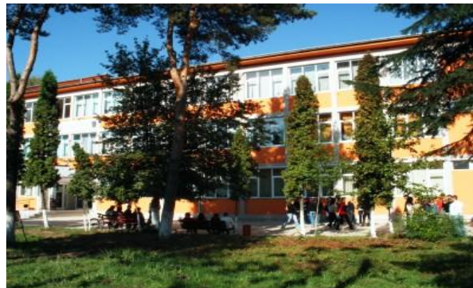
North Center University Baia Mare, Romania
